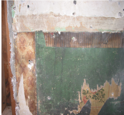
Layers of paint and wallpaper in the kitchen, 19 th and 20 th centuries.
